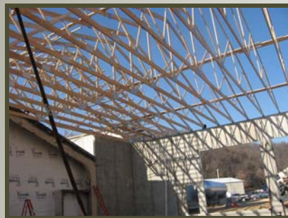
Rafters Set in Place
