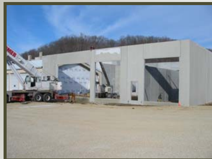
Completed Panel Installation
