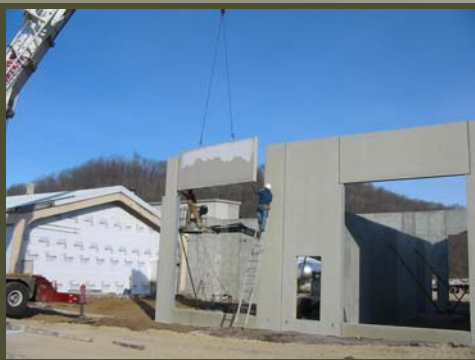
Setting Cross Beam
