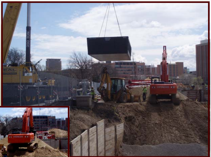
Above Setting Bottom Tank Section
