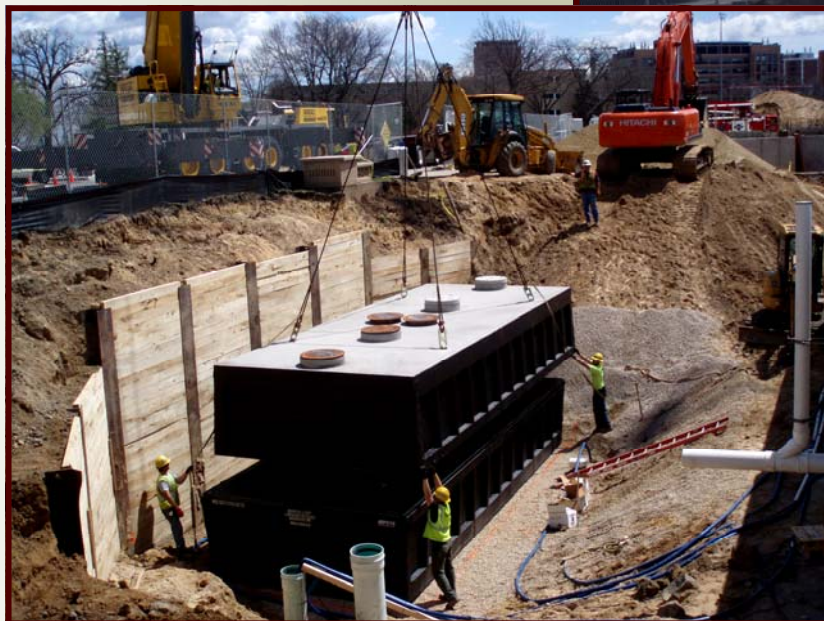
Above Setting Bottom Tank Section
