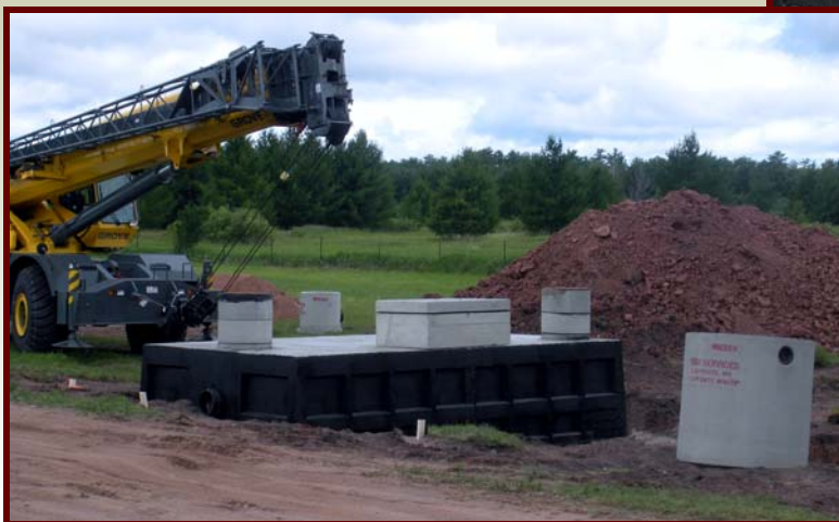
Left: Tank Installation Completed
