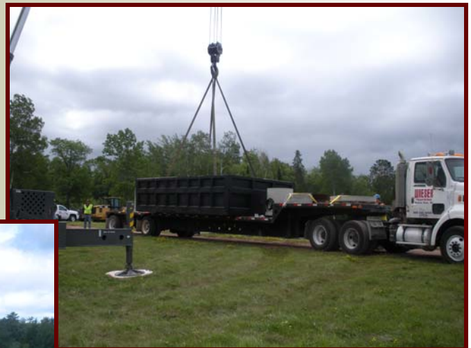
Above: Unloading Bottom Section of 12,000 Gallon Capacity Precast Tank
