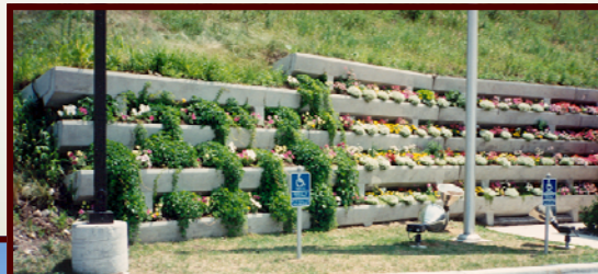
Evergreen Retaining Wall
