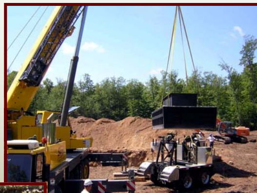
Above: Crane Setting Tank.
