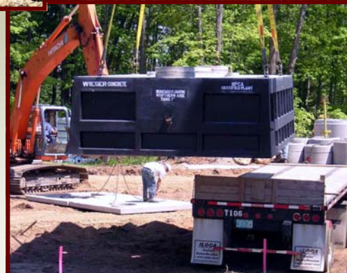
Below: Crane Lowers the Upper Section of a FAST System Tank in Place.
