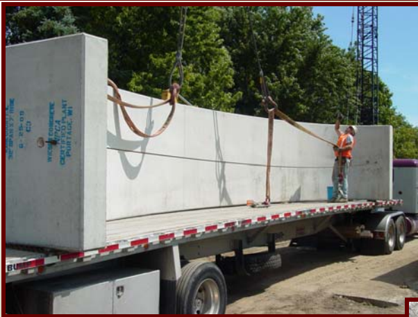
32' x 7' Bridge Section being unloaded at jobsite.
