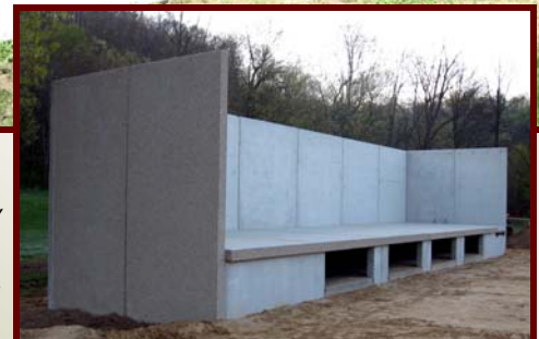
Right: Back wall and stage completed.
