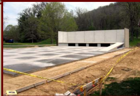
Right: Project is ready to be completed. Precast building panels, and handicap ramp are in place and concrete floor is complete.
