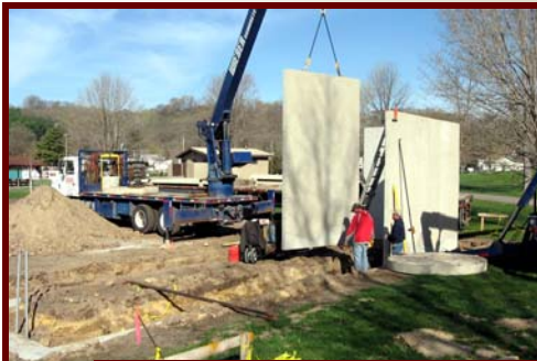
Left: Setting Stage Back Wall with Exposed Aggregate Building Panels
