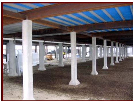
Storage Area Beneath Slatted Pit Top
