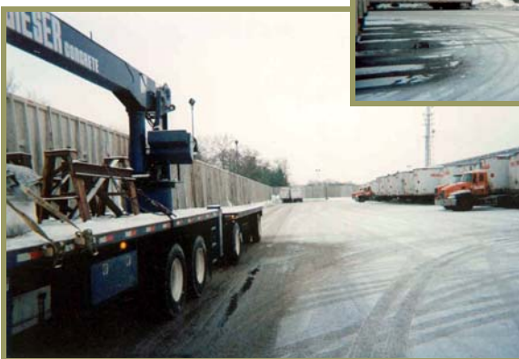
Completed Noise Wall
