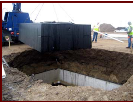
Setting Top Section of Grease Interceptor
