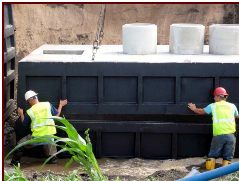
Setting Top Section of 7700 Gallon Tank
